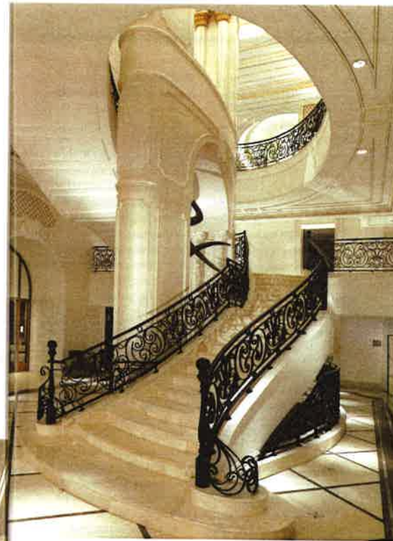
The entrance lobby features a grand staircase that is clad in marble and has an intricate ironwork railing. The central, decorative arch conceals the concrete column from which portions of the stair cantilever 1.5 m.
